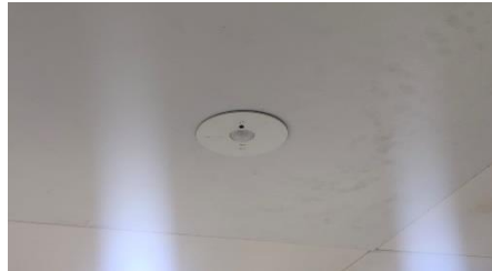
Motion Sensor for Restroom Lighting Control
