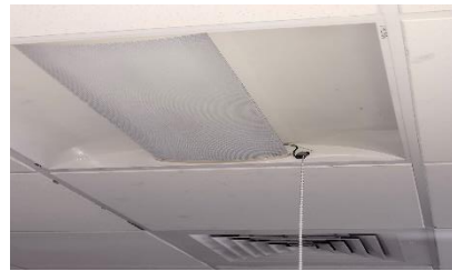
Pull Cord Switch Installation for Lighting
